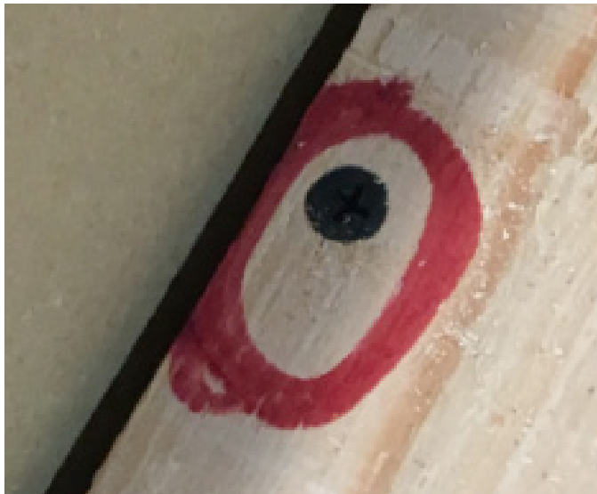
FIGURE 1— Remove the Phillips head screw on top of the side supports.
